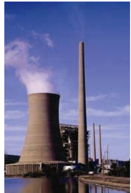
Buckeye's Cardinal power plant has had nearly $900 million in environmental upgrades.
